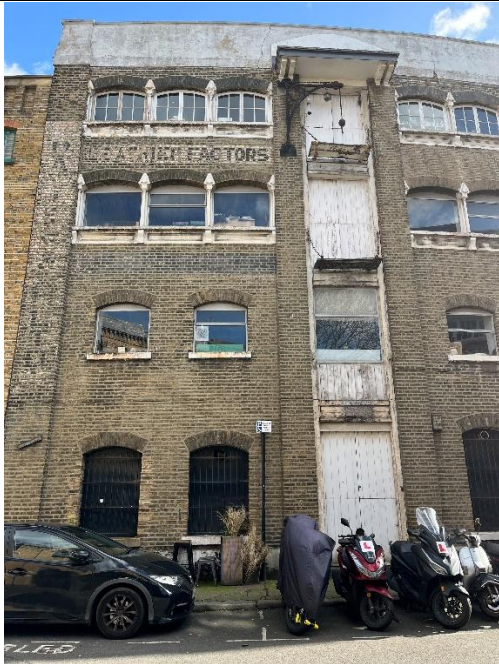
A yet to be refurbished warehouse
